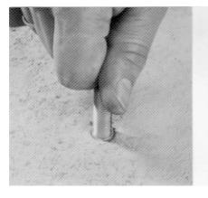
Screw the threaded rod in internally threaded anchors such as the HKD (HDI) or TDD (HSS). In the case of the HSL replace the bolt by the threaded rod.
